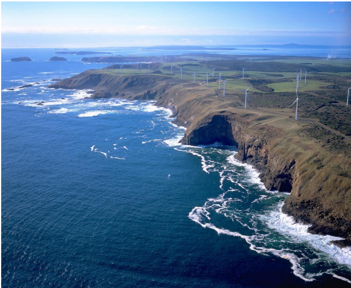
Figure 1. A coastal view of the 140 MW Woolnorth Wind Farm, located on the far north-west coast of Tasmania where the Great Southern Ocean meets Bass Strait. Up until April 2008, this was the biggest wind farm operating in the southern hemisphere.
